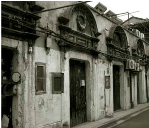
Top: Shanghai's French concession. Photo: Liu Gang Below: Typical lilong house. Photo: R. Mason/PennDesign
